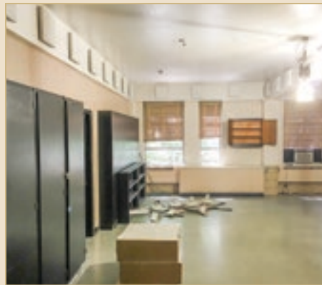
Renovations underway this summer in the St. Joseph classrooms.
